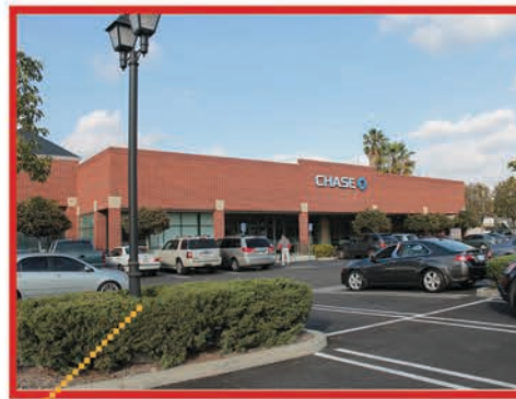
View northeast towards Chase
