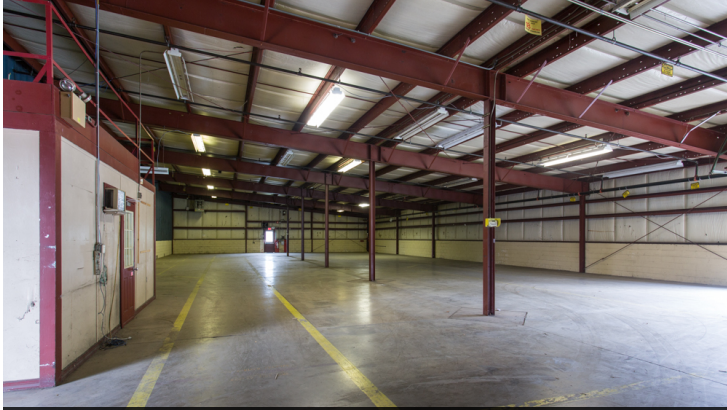
7800 SF shipping warehouse
