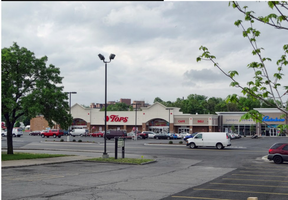
CENTER: VIEW FROM EAST RIDGE ROAD
