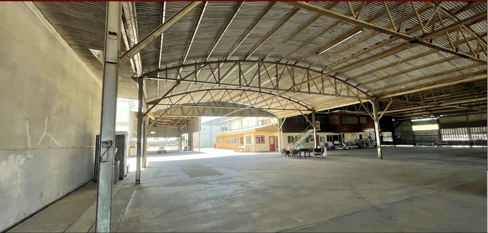
Warehouse G View of covered entrance and outside entrance
