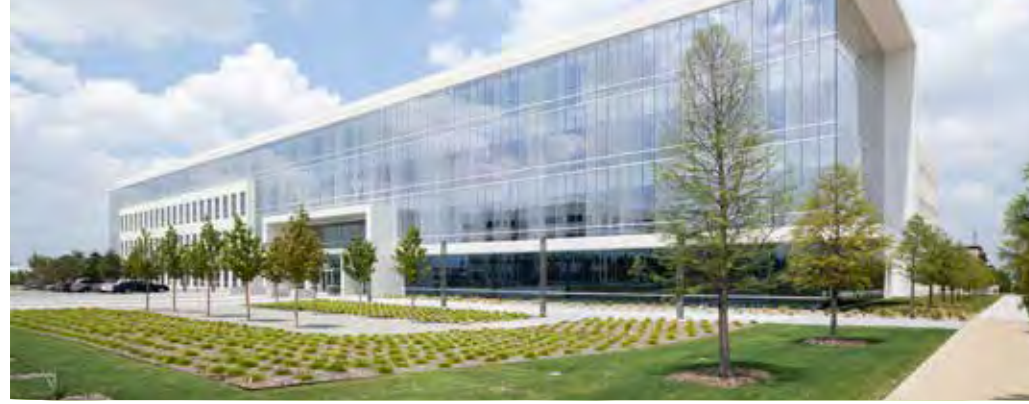
9111 CW Blvd - Spec Building
