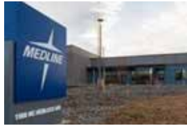
Medline Renewal Building -Photo Courtesy: Tim Paik
