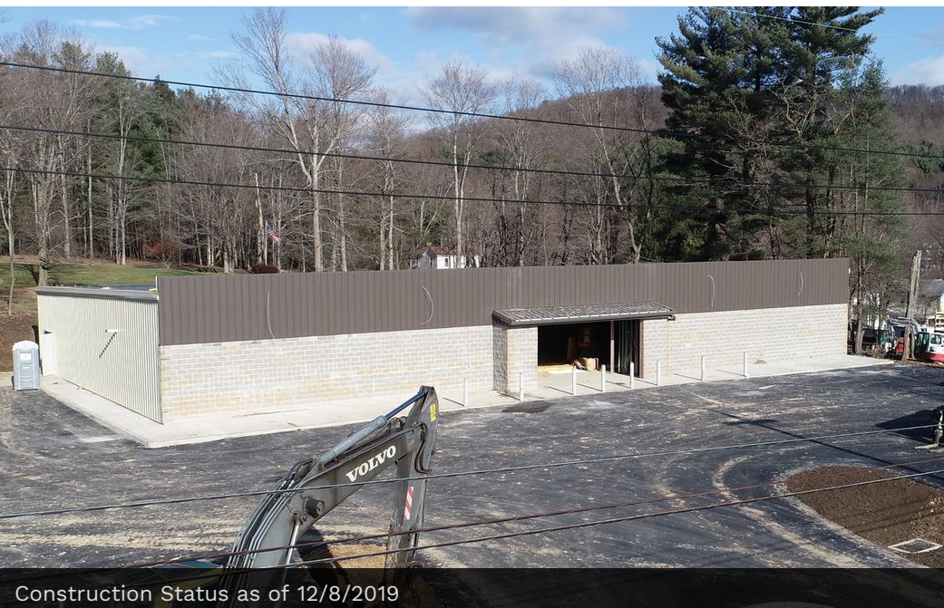
Construction Status as of 12/8/2019
