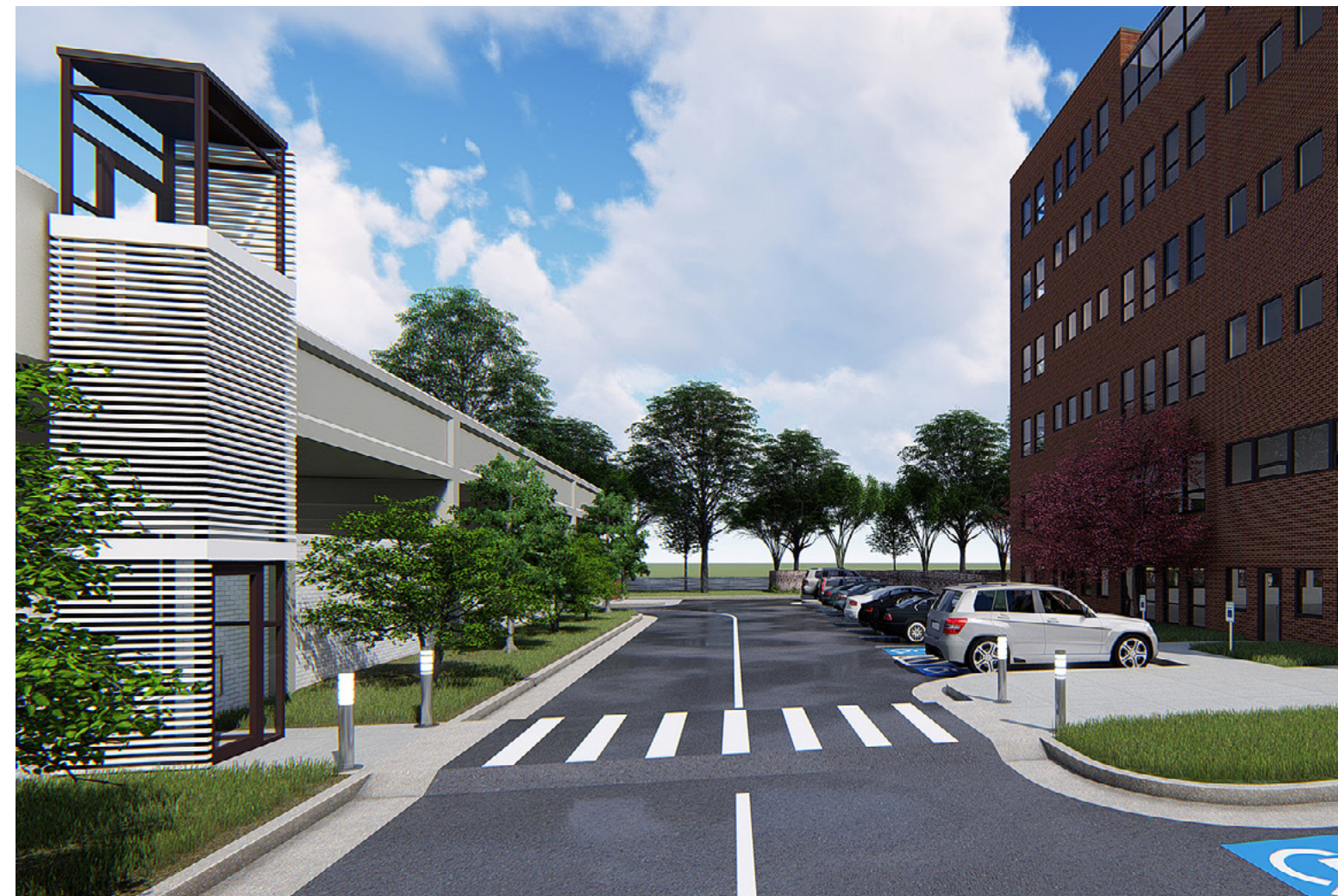
Brand new parking elevator
