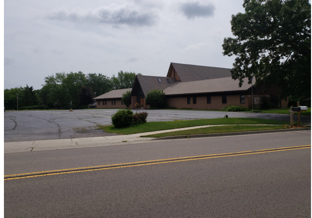
Side Exterior View
