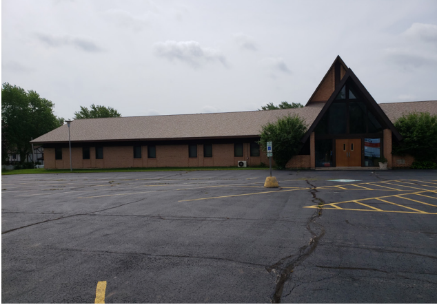
Side Exterior View
