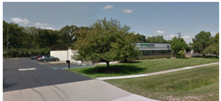
Building Exterior & Parking
