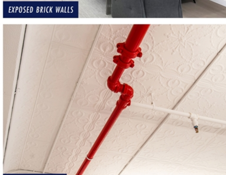
EXPOSED BRICK WALLS
