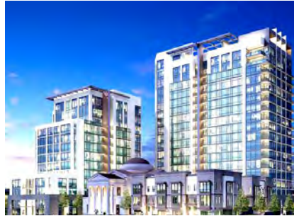
Parkview Towers - 220 Residential Units and 18,000 SF Retail
