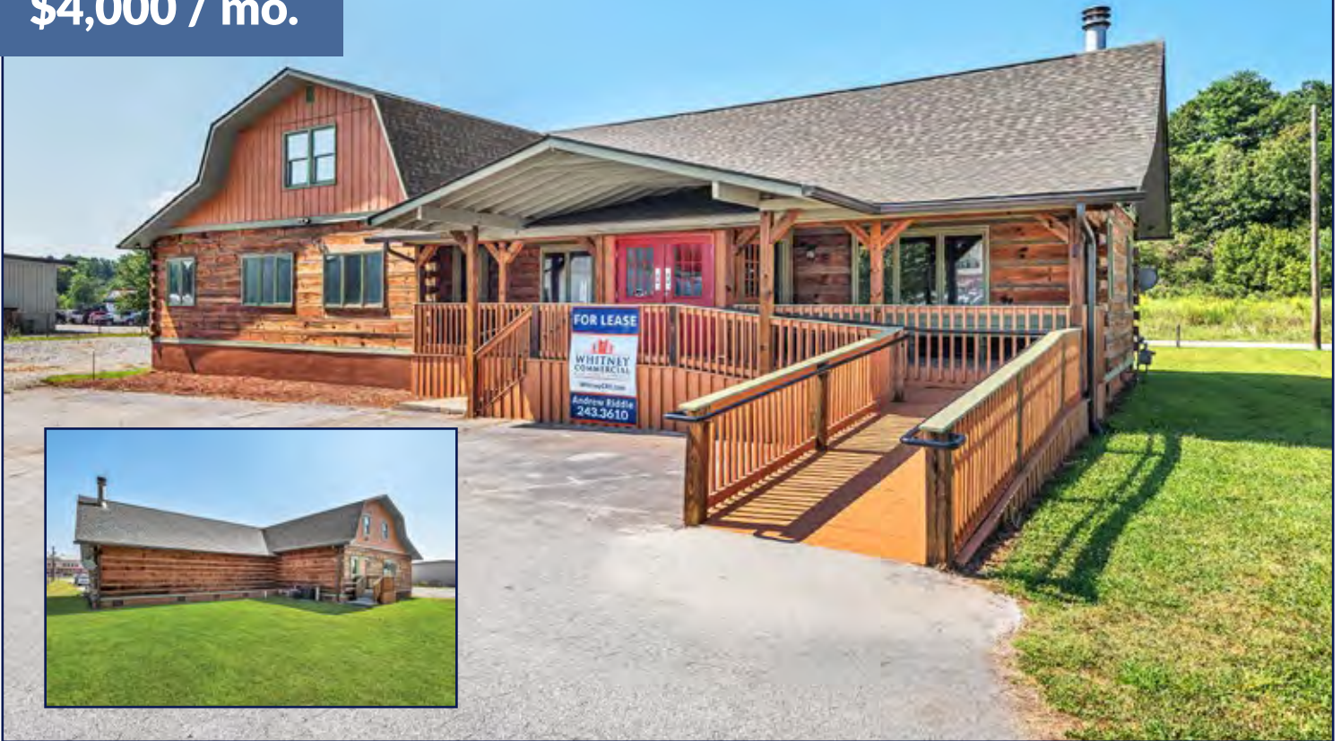
Front of building showing accessibility ramp; Inset: Rear exterior
