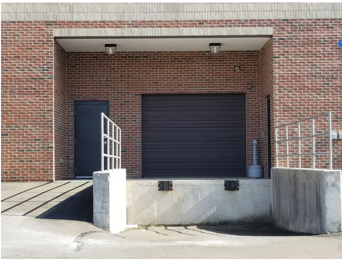
Dock High Loading Dock
