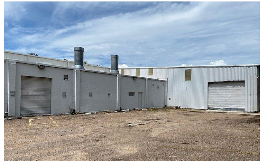
Two grade-level entrances to the manufacturing space
