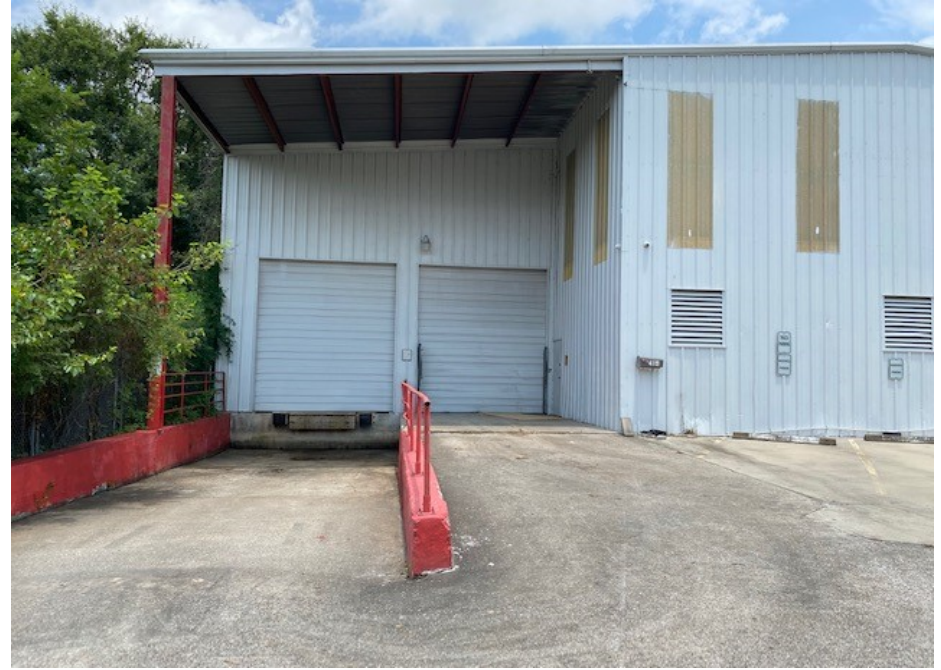
Covered delivery capabilities
