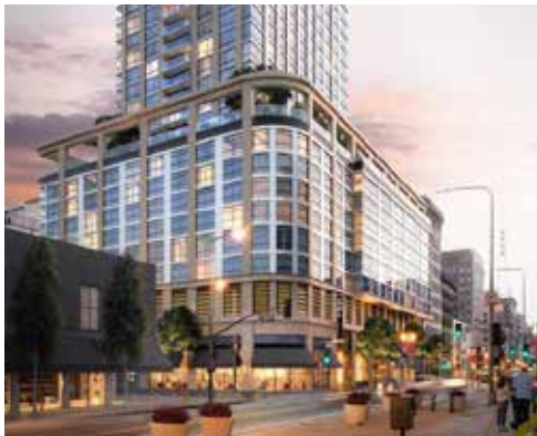
UNDER CONSTRUCTION PERLA
