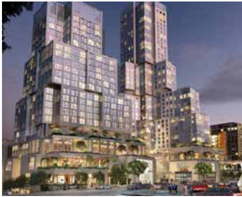
UNDER CONSTRUCTION THE GRAND
