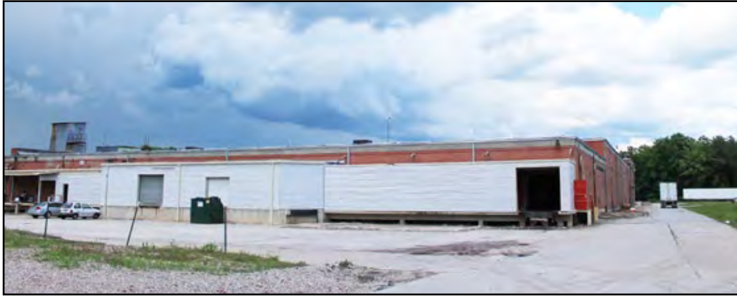
Main Building - Back side with dock-high doors and loading doors
