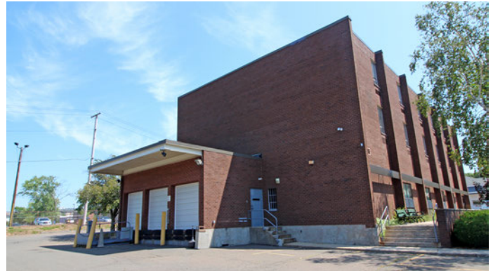
THREE LOADING DOCKS
