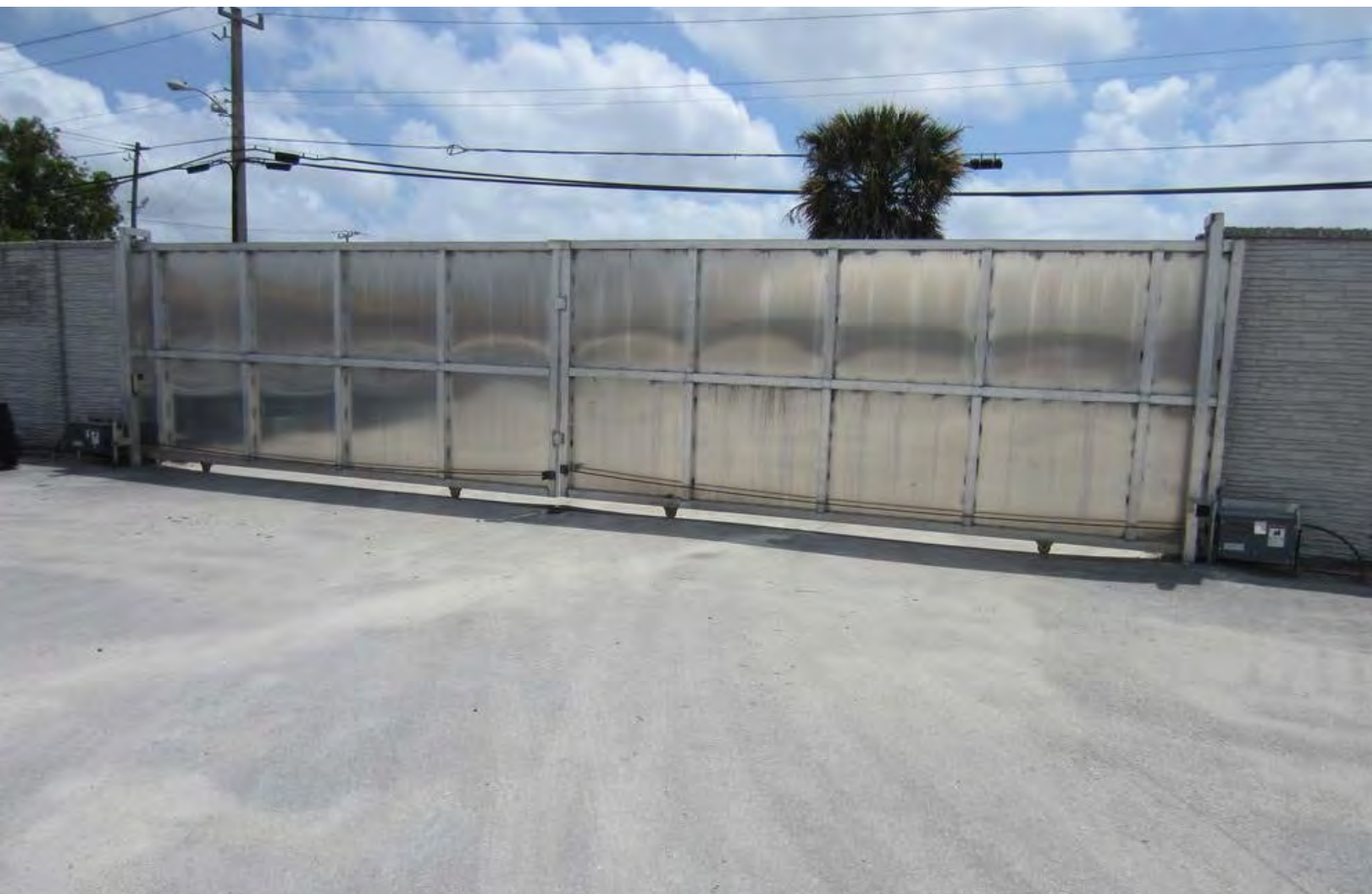
Motorized Steel Gate Entrance into Yard
