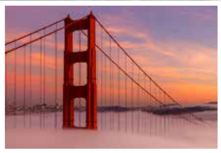
GOLDEN GATE BRIDGE
