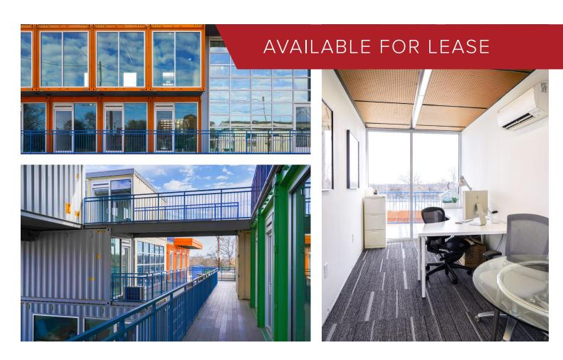
Three story office/retail building developed using 40 shipping containers. Each shipping container is 8 feet by 20 feet and 1 foot taller than the typical container size. Each office is approx. 160 square feet and ideal for one person. The building will have a break room, restrooms, common areas, as well as solar panels and wind turbines to generate supplemental power for the offices.
