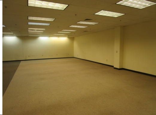
Photo 34: View of interior suite on ground floor
