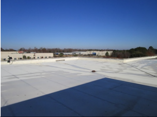
Photo 19: View of northwest portion of roof
