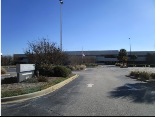
Photo 1: View of building facing east
