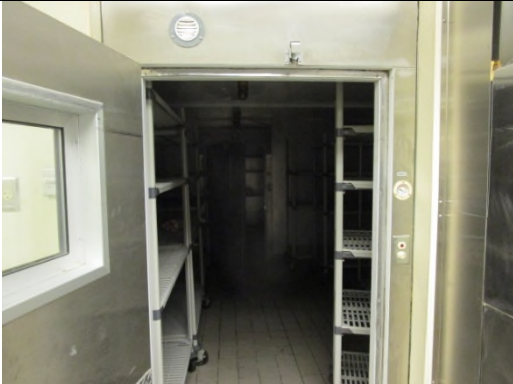
Photo 45: View of walk-in cooler in ground floor kitchen
