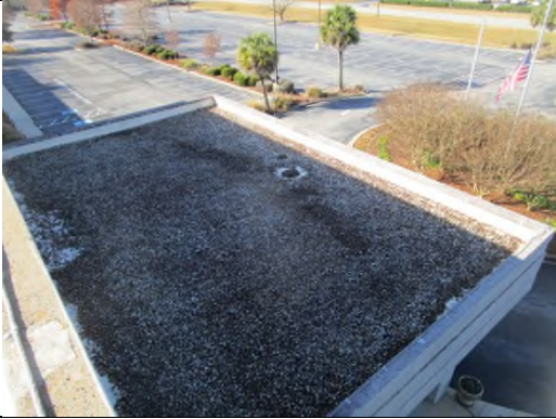
Photo 17: View of roof over west entrance canopy
