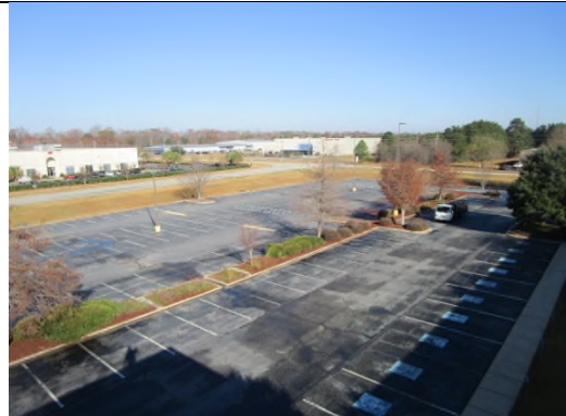
Photo 14: View of west parking lot facing northwest
