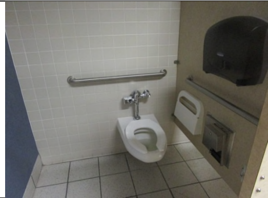
Photo 42: View of handicap accessible toilet in ground floor restroom
