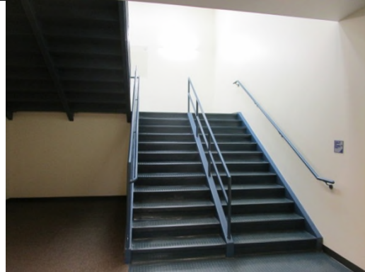
Photo 28: View of stairwell at lobby area
