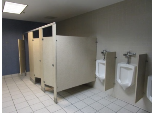
Photo 52: View of second floor men's restroom
