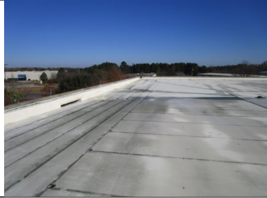
Photo 18: View of roof facing northwest
