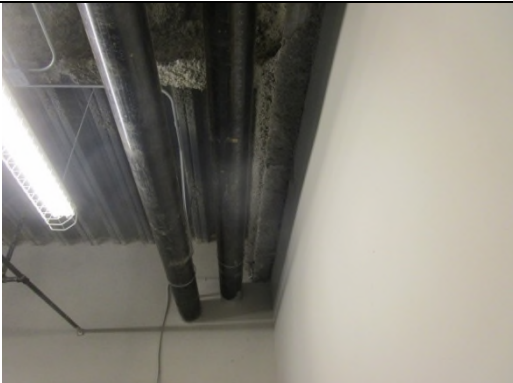
Photo 29: View of exposed building framing with sprayed fire proofing
