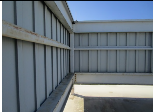
Photo 24: View of RTU screen wall (typical)
