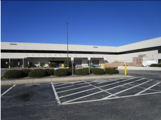
Photo 5: View of east loading dock area
