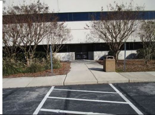
Photo 4: View of south entry of building
