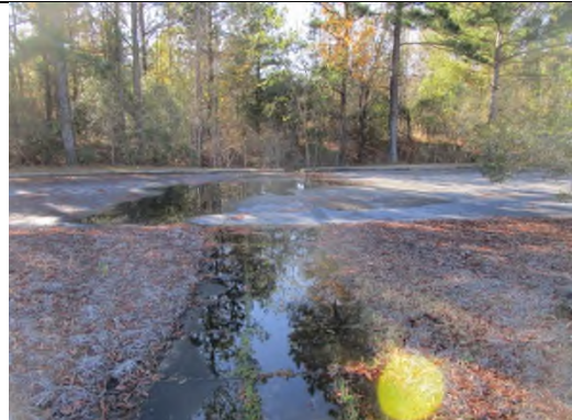
Photo 8: View of poor drainage conditions at south perimeter drive
