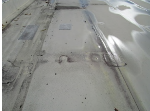
Photo 20: View of debris at roof drain
