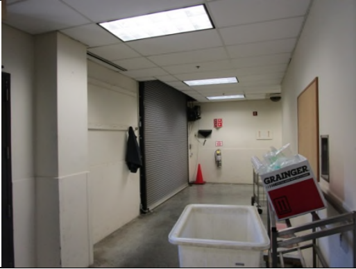
Photo 49: View of loading dock on east side of building
