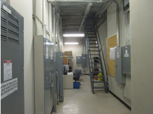
Photo 27: View of electrical room and roof access
