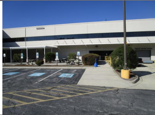
Photo 10: View of handicap accessible parking stalls at east side of building
