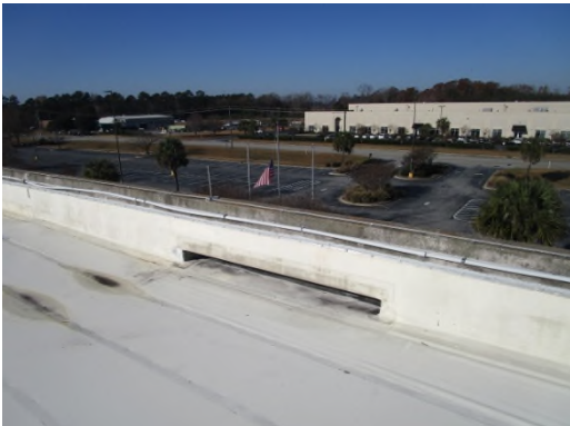
Photo 21: View of perimeter roof scupper
