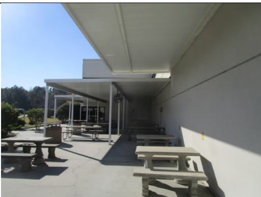
Photo 15: View of patio at east side of building
