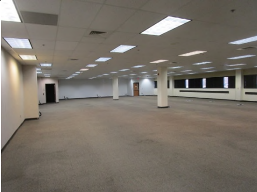
Photo 37: View of north open office area on ground floor
