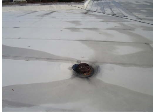
Photo 20: View of debris at roof drain
