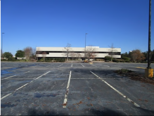
Photo 3: View of building facing north
