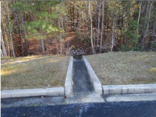
Photo 7: View of drainage flume at east side of site
