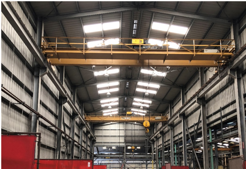
Twelve cranes throughout the building Steel framing is hot dipped galvanized
