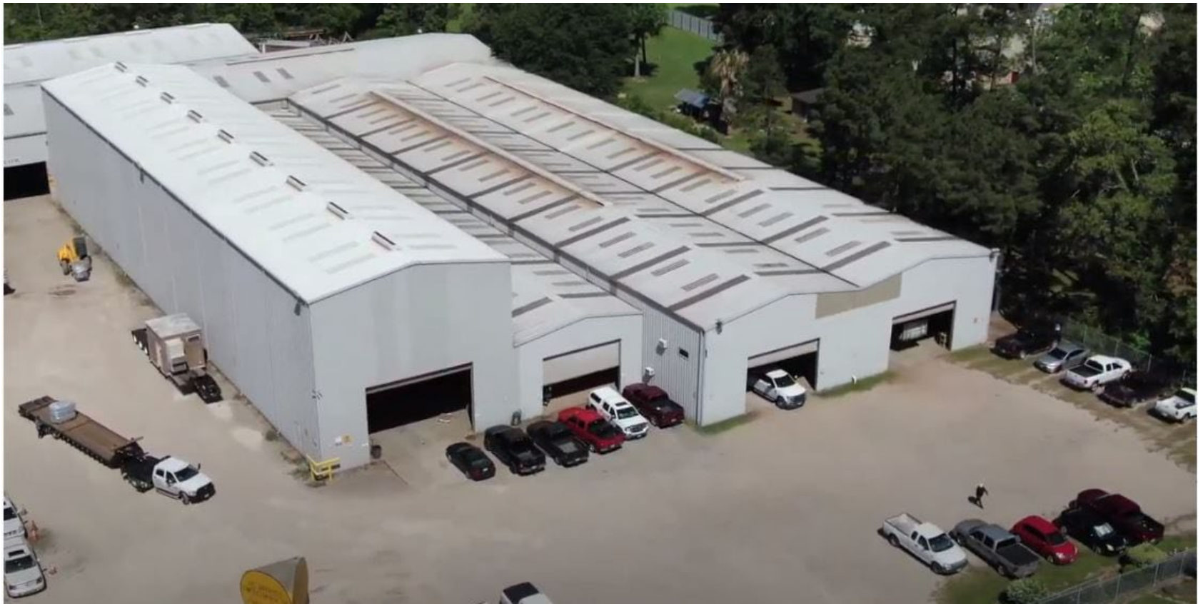
Four long bays with two perpendicular cross bays at the rear
