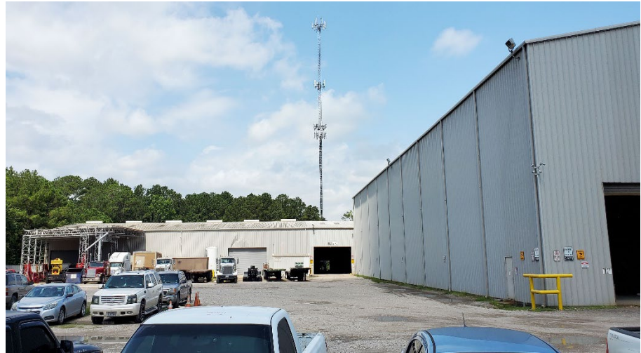
Perpendicular cross bays at back
