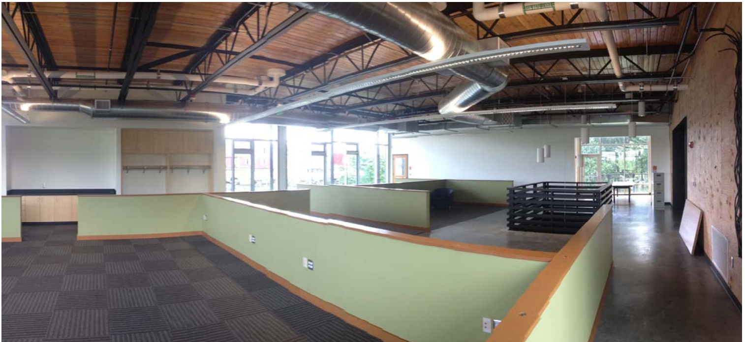
Polished sealed cement floor, carpet tiles within built-in partitions, open ceiling, small break area.
