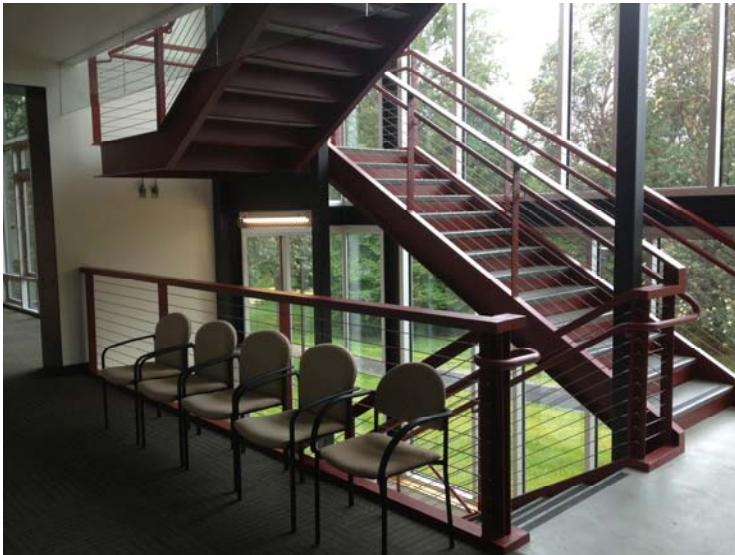
Main staircase to all levels, with elevator to the right
