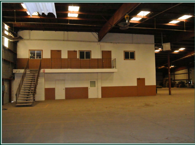
Interior of 22,000± SF warehouse. 6 interior offices and 4 loading docks.
