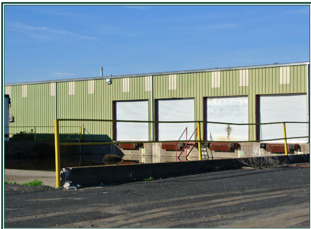
Exterior of 22,000± SF warehouse. 4 roll up doors.
