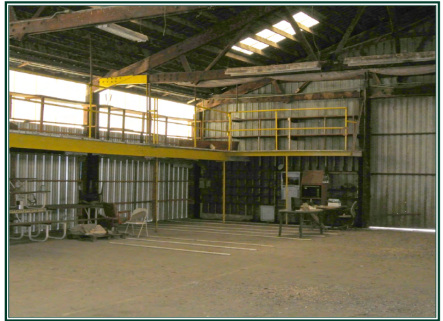
Interior of Shop. 2 roll up doors, 2 large sliding doors.
