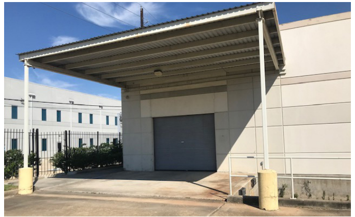
Dock and drive-in at overhead door
