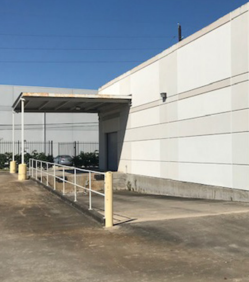
Covered delivery dock
