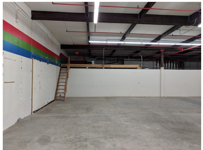
Warehouse and mezzanine
