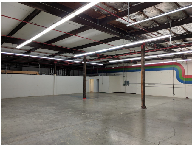
Warehouse and entrance from offices
