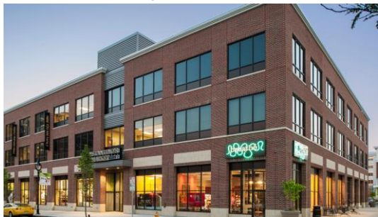
Night Scope – Building 3
