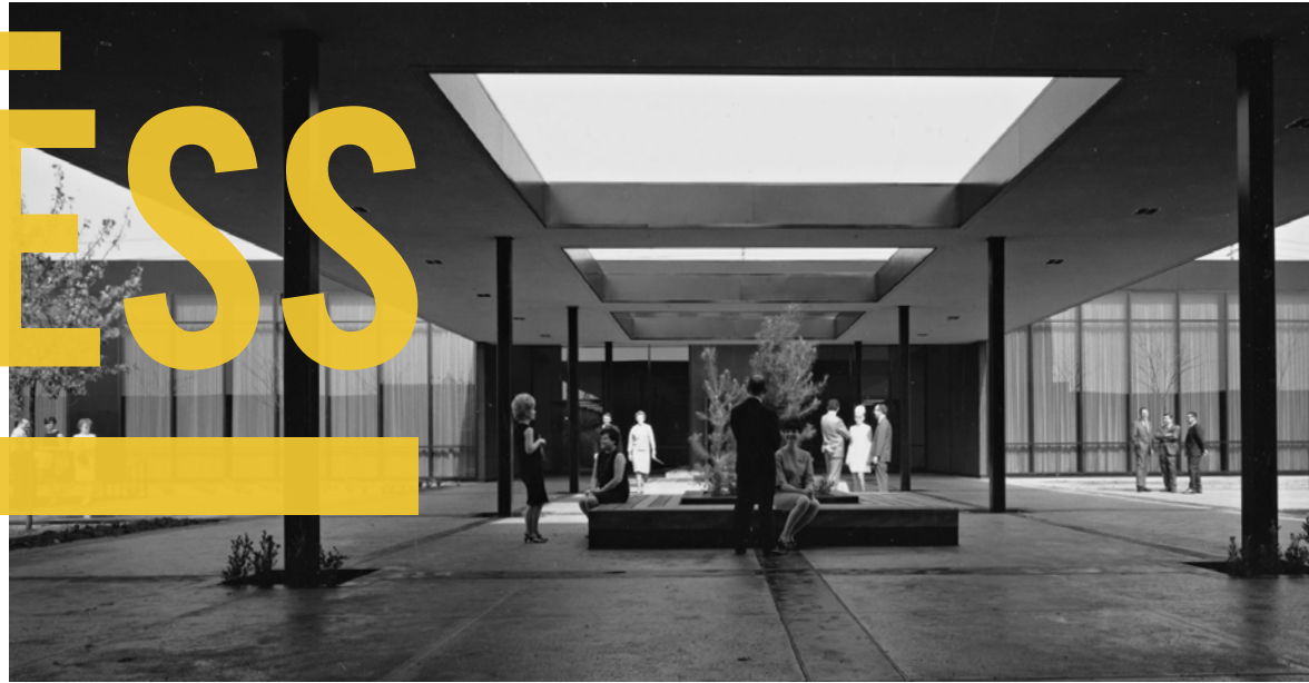
The press facility in 1968. Courtesy Costa Mesa Historical Society.
