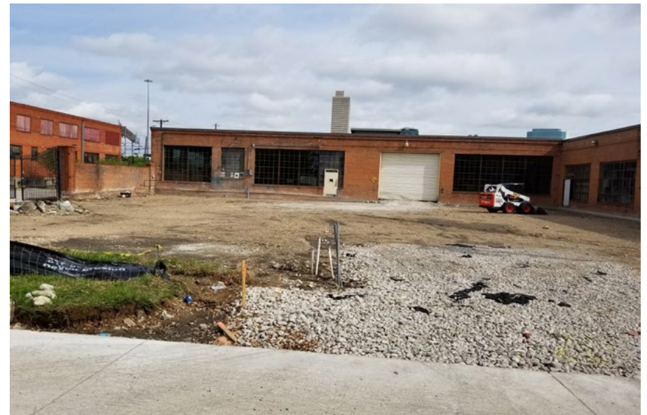
* BACK PARKING LOT CONSTRUCTION UNDERWAY
