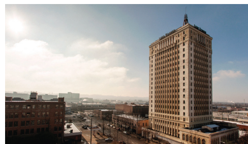
Thomas Jefferson Tower
