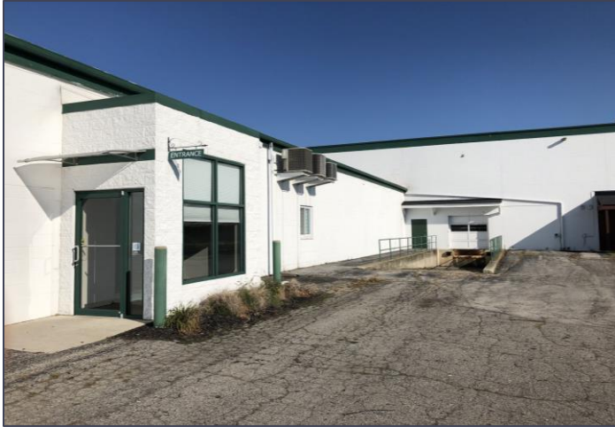
Front entrance and dock
