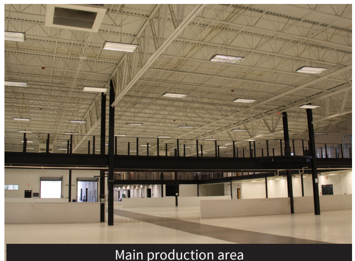
Mezzanine / catwalk in main production area
