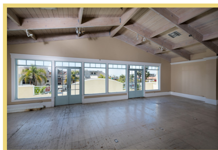
Second Floor Street-side
