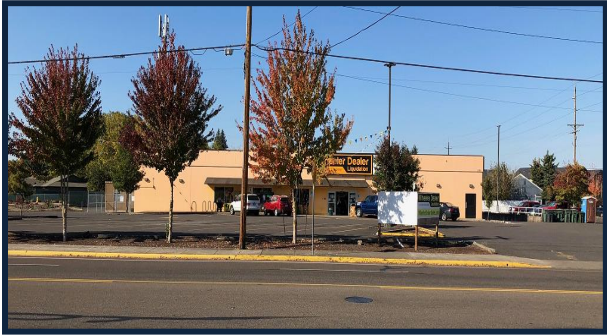
The building faces Geary Street. Loading dock located on right.
