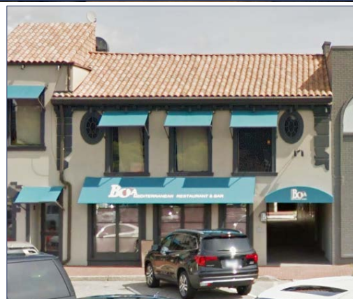
Entrance from Parker Harding Plaza
