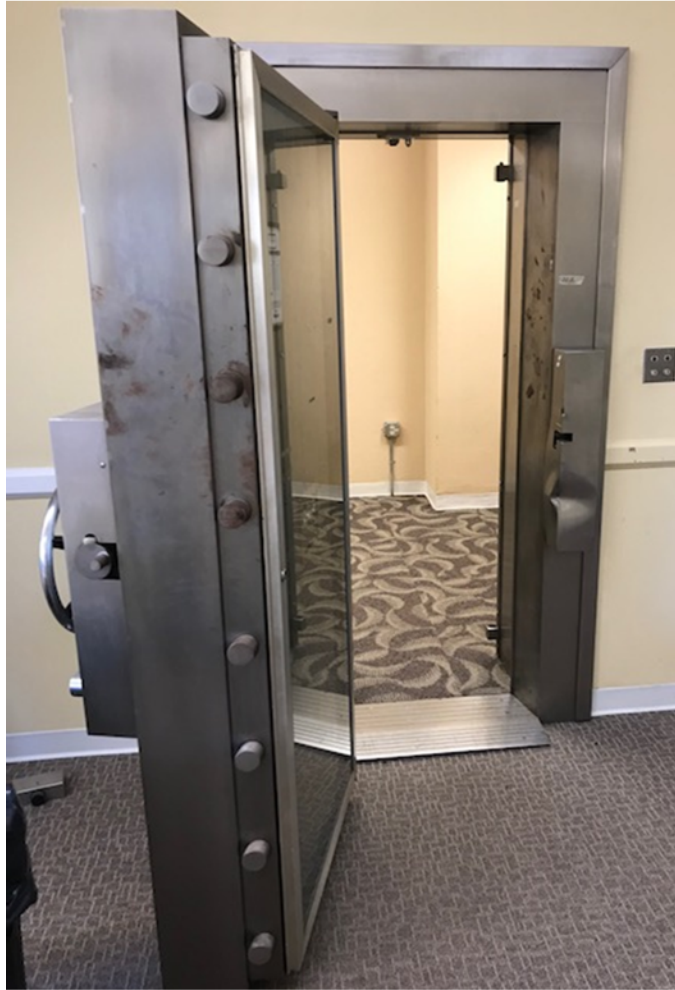
First Floor Vault (Office Conversion)
