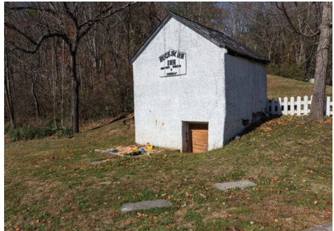
Additional Storage Area
