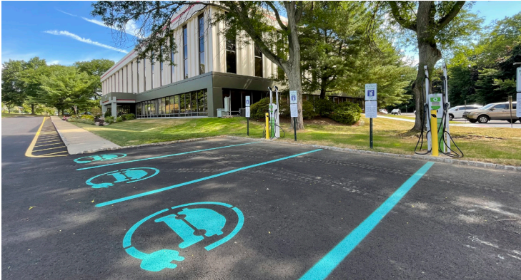
New EV Charging Stations
