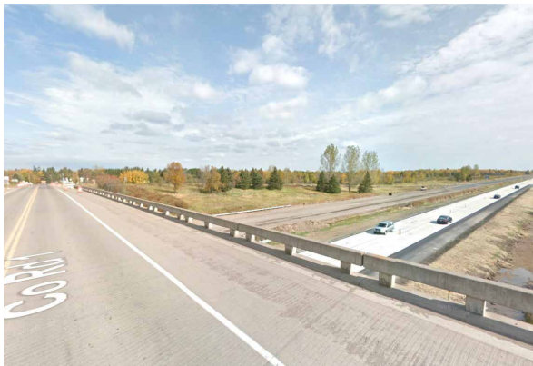
Thomson Road Overpass Looking Northeast
