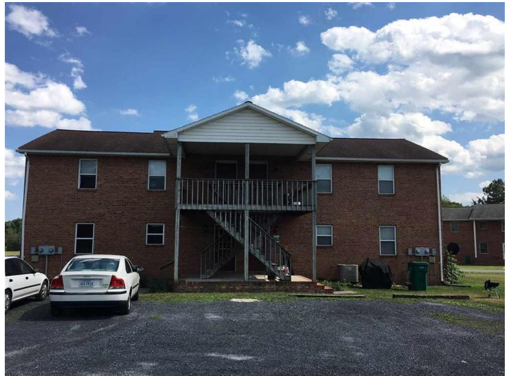
Back View of Building w/ Gravel Parking Area
