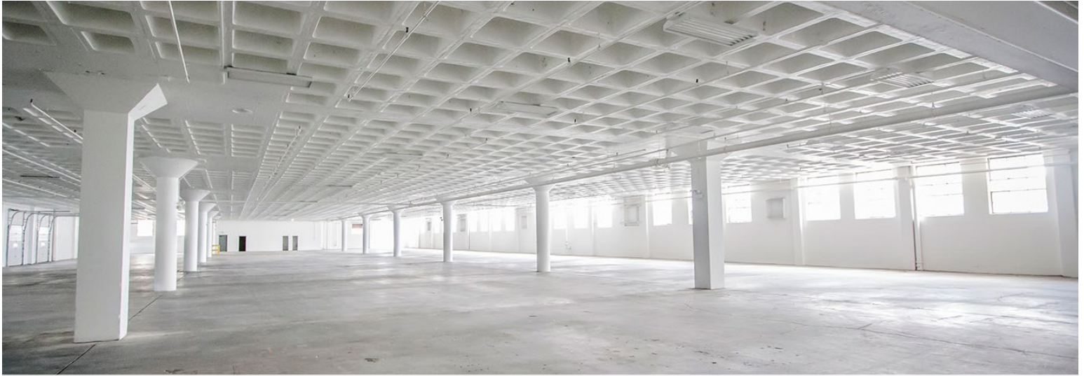
First Floor Interior
