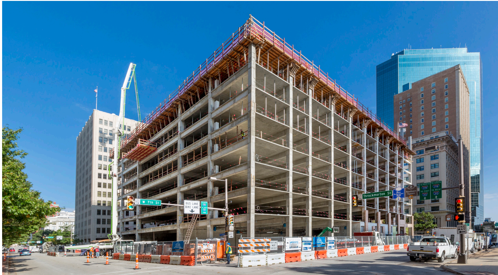
CONSTRUCTION PROGRESS as of NOVEMBER 18, 2016.
