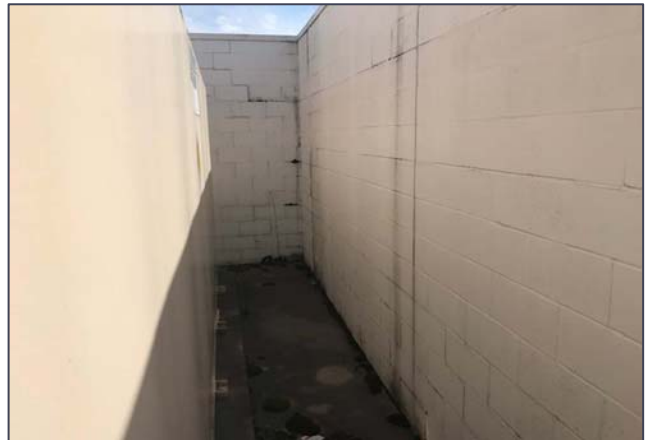
Fuel tank protective wall
