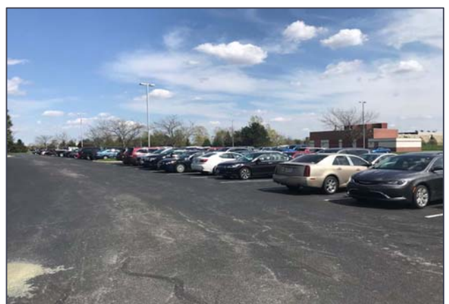
Rear parking lot
