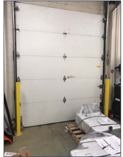
Main level 10' warehouse door for deliveries
