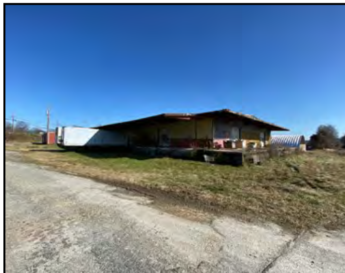
Exterior: loading dock area
