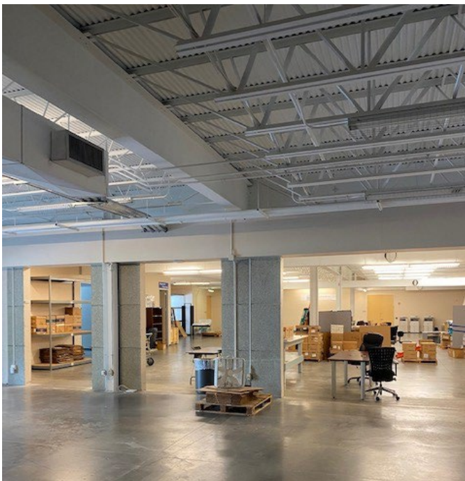
Openings to original building from expansion
