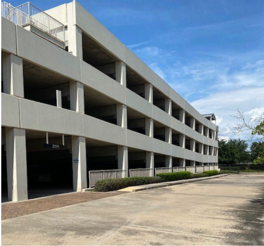
Parking garage serves both buildings providing 269 spaces
