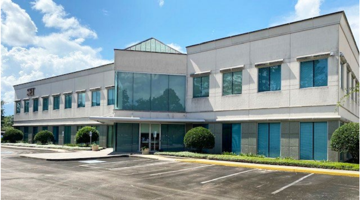
Steel structure with custom tiltwall panels
