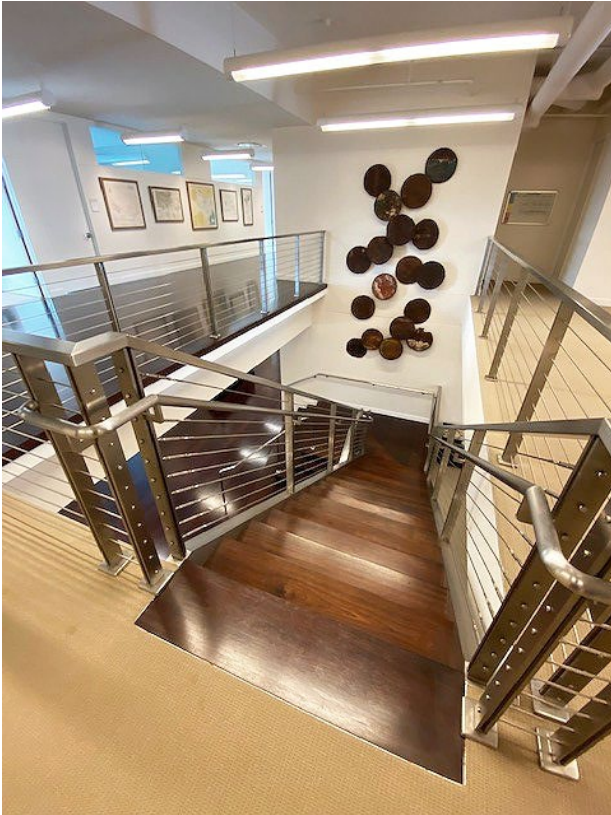
Internal staircase between Levels 4 and 5
