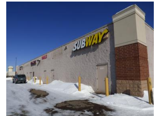
Rear of Building
