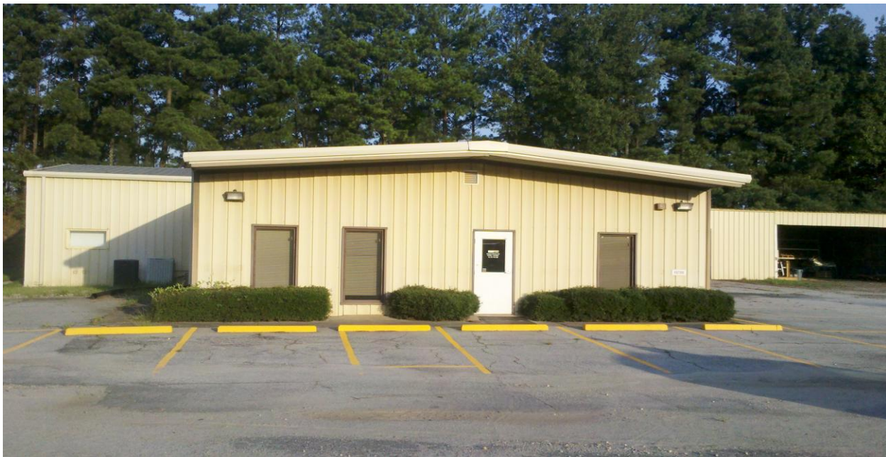
Front of Office
