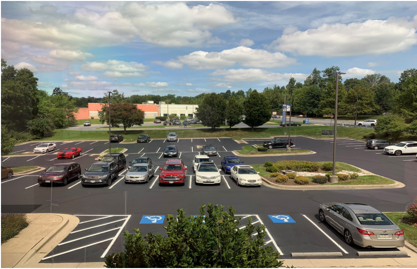
North West View of Parking Area
