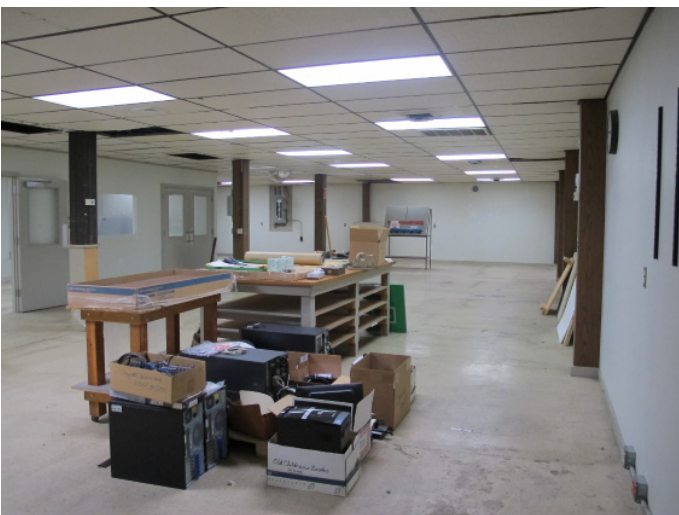
Middle area - formerly prep room
