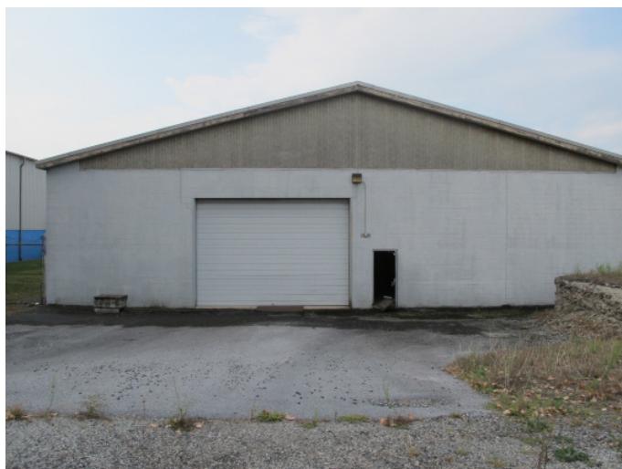
At grade door (exterior-rear)
