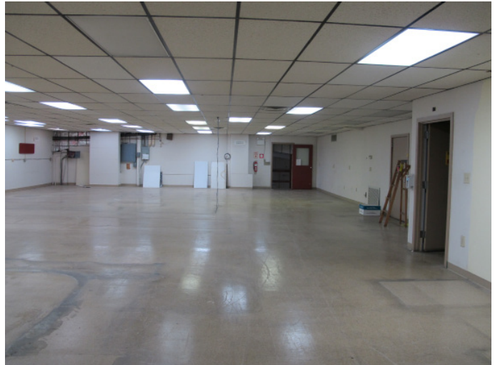
Second level mezzanine
