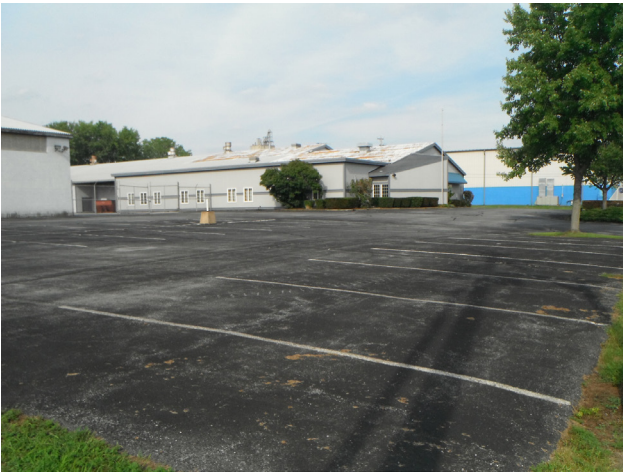
West side exterior of offices
